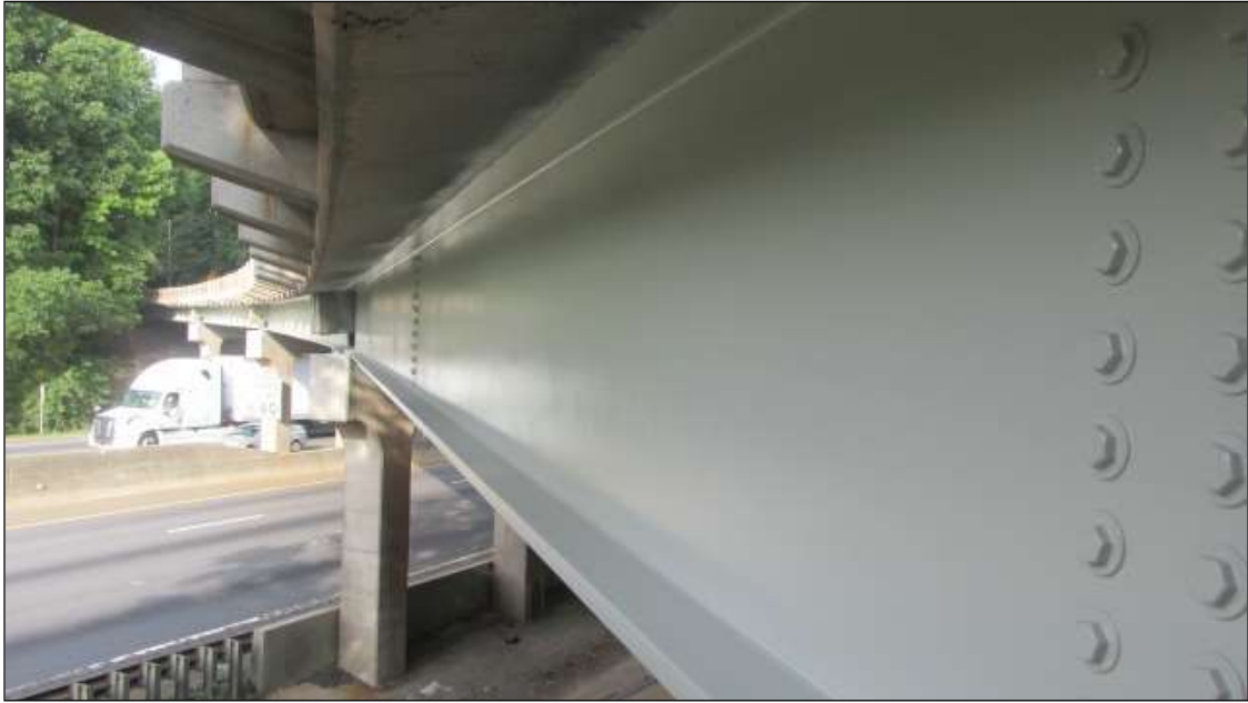
BMS., BEARING AND DIAPHS PAINTED- COATING I
