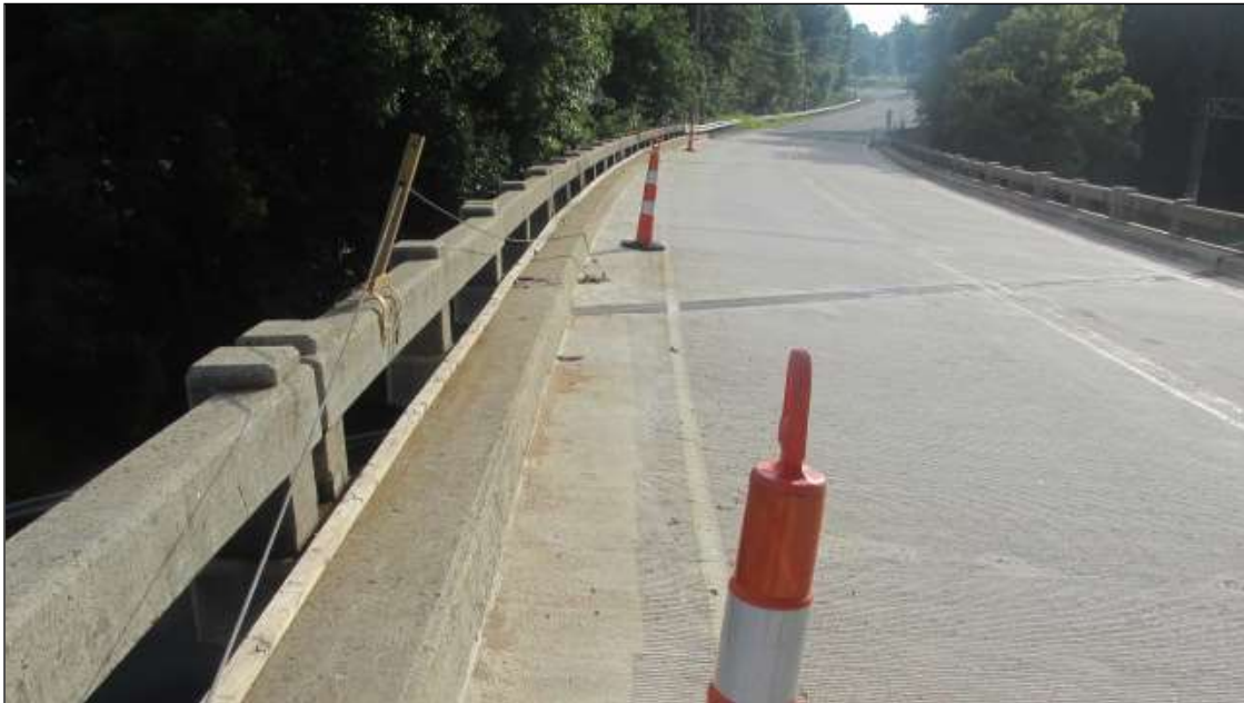
PHOTO SHOWING CONES AND CABLE ALONG THE RAILS STILL IN PLACE
