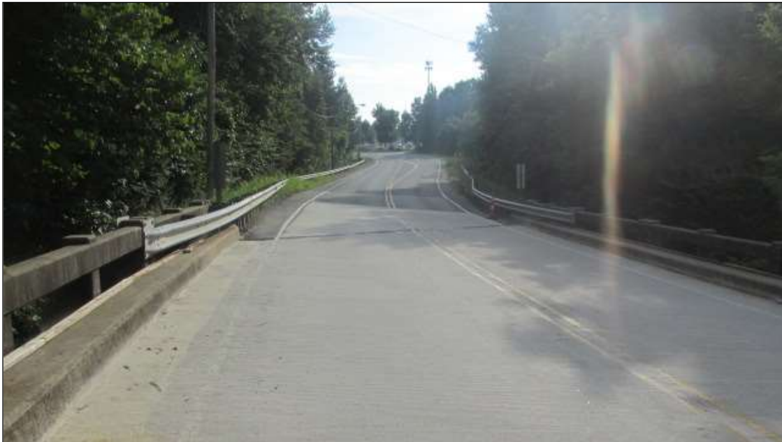
GUARDRAIL LOOKING EAST
