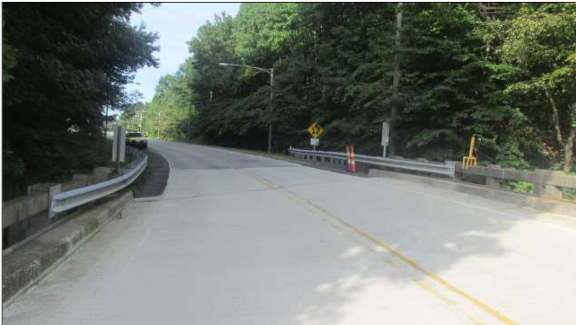
GUARDRAIL LOOKING WEST
